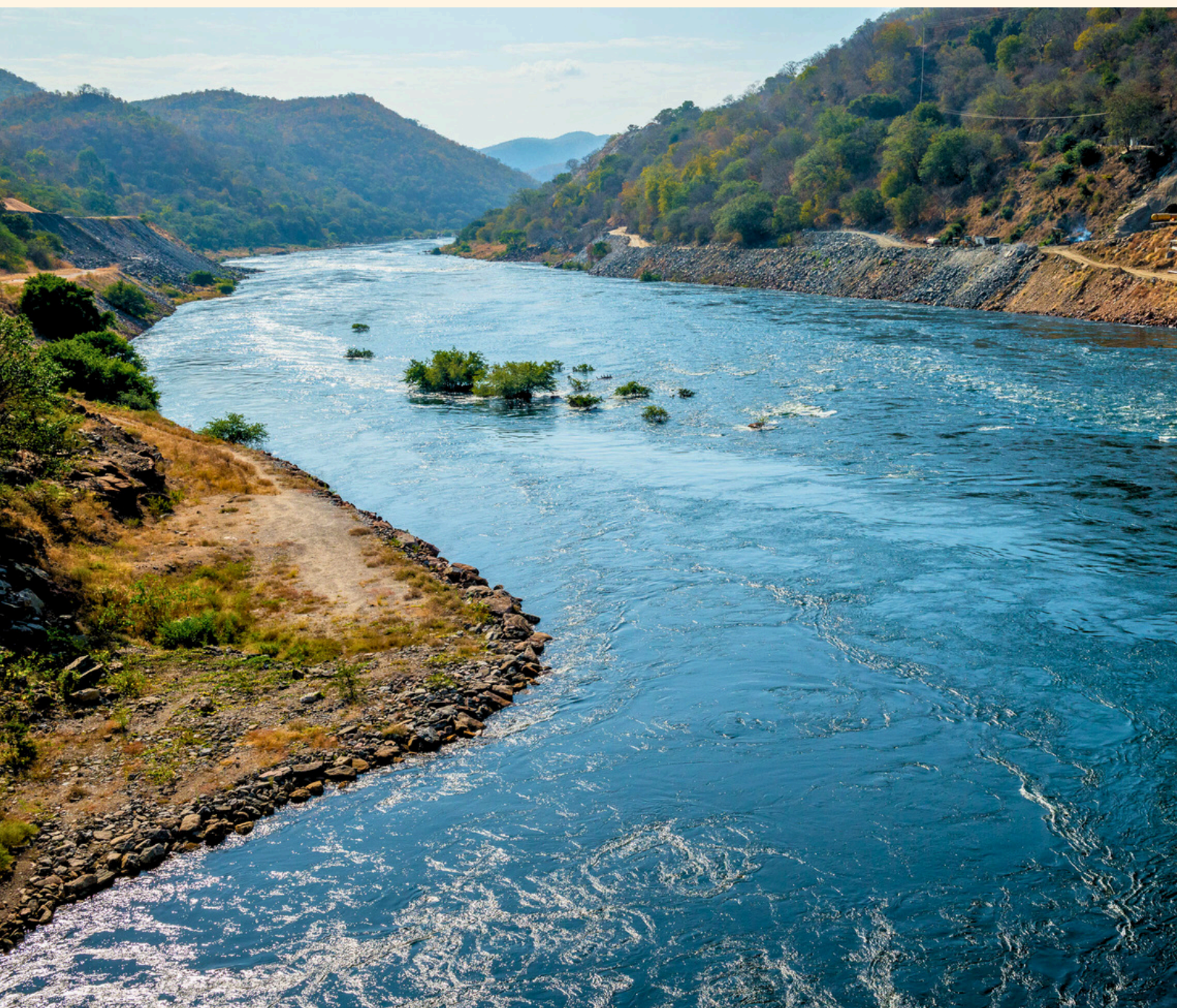
Earthworks on the banks of the Zambezi River, Zambia. ©Arne Hoel
