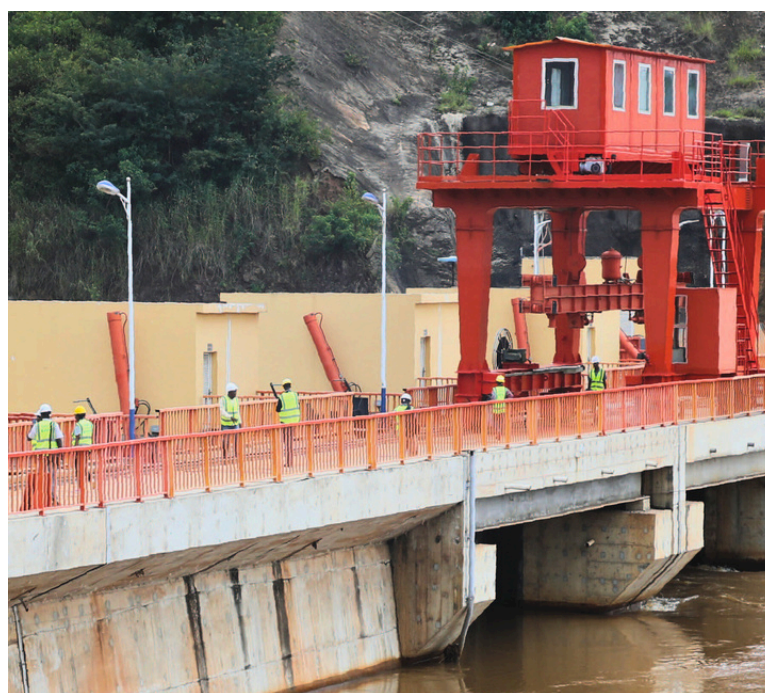
Regional Rusumo Falls Hydroelectric Dam, Rusumo, Tanzanian-Rwanda border. ©NBI
