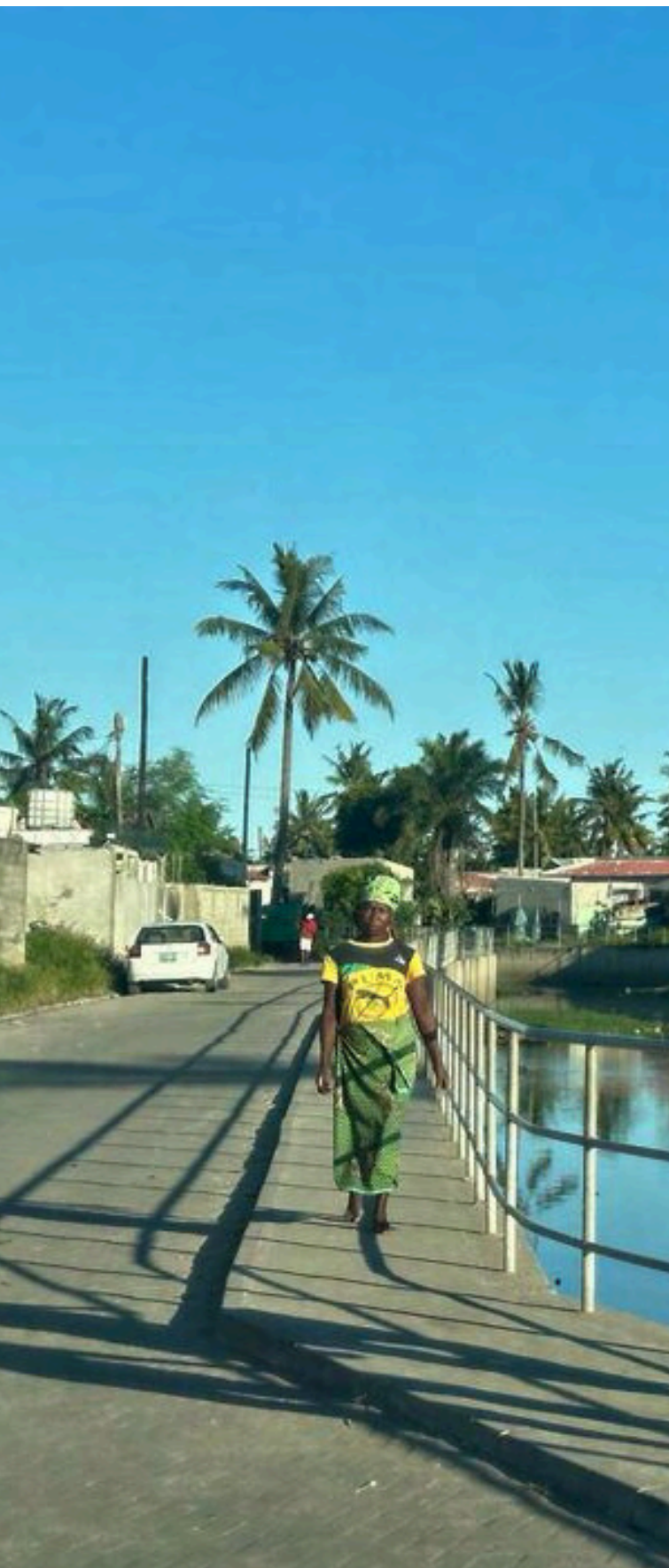
Woman walking next to the storm water drainage system, Beira, Mozambique. ©Franka Braun / World Bank
